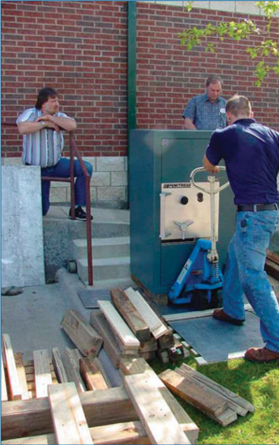
4. Starting the cribbing at the bottom step.
